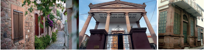
Figure 10: Use of sarımsak taşı in load-bearing elements
