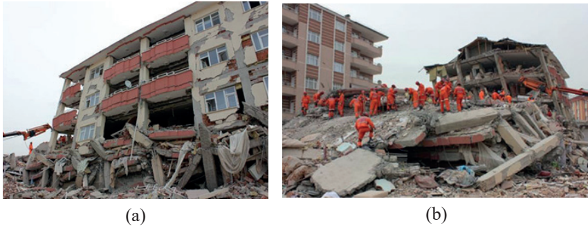
Figure 5. 2011 Van earthquakes; (a) soft storey irregularity, (b) inability of the building structure to withstand earthquake loads (Damcı et al., 2015)
