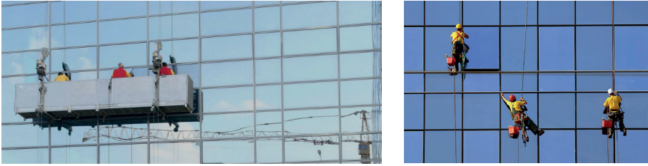
Figure 1. Cleaning of high-rise building façades with traditional methods (URL-1; URL-2)
