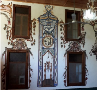
Photo 9: Kırkoluk Mosque, last congregation place, west part, south wall outer mihrab (Photograph taken by Başak Katrancı, 2017)
