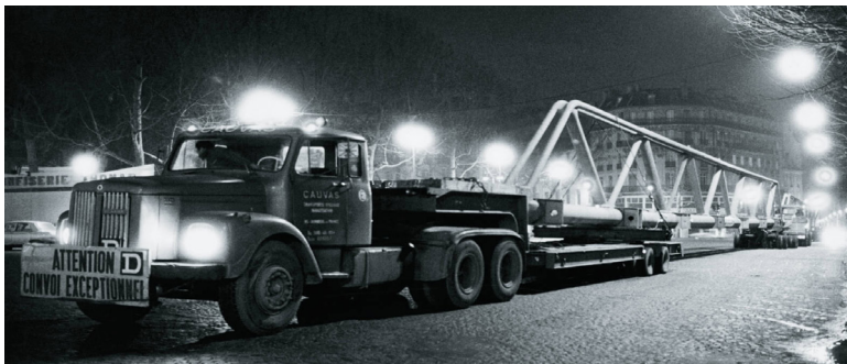
Figure 10. Transport of prefabricated elements to the construction site during the construction phase of Center Pompidou ( https://rshp.com/projects/culture-and-leisure/centre-pompidou/access date: March 2024)
