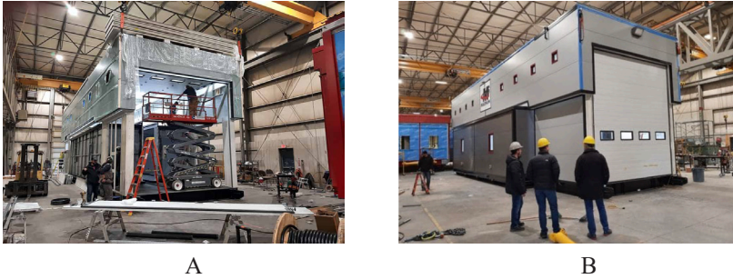
Figure 17. Prefabricated fire station with all systems produced in a factory environment
