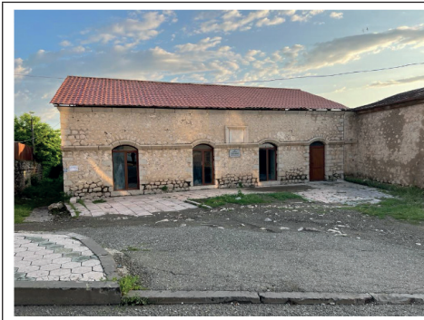
Photo 3. Mamay Masjid, south facade.
