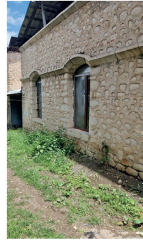
Photo 4. Mamay Masjid, west facade.
