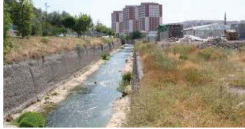
Figure 9. Urban transformation project on Hatip Stream, Mamak ( https://www.evrensel.net/haber/32937/hatip-cayinda-tehlikeli-donusum )
