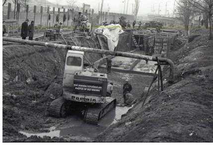
Figure 23. Covering works of Incesu Stream, 1960 ( https://www.pinterest.de/pin/535787686909925999/ )
