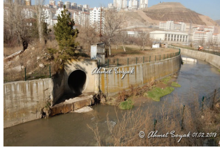
Figure 6. Hacıkadın Stream in the channel, 2018 (Soyak, 2018)
