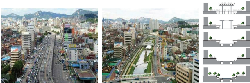
Figure 43. Cheonggyecheon Stream Restoration Project: Before and After Transformation Photos - road demolition and stream restoration procedure (Liste List, 2017) (Seo and Kwon, 2018, p.4)
