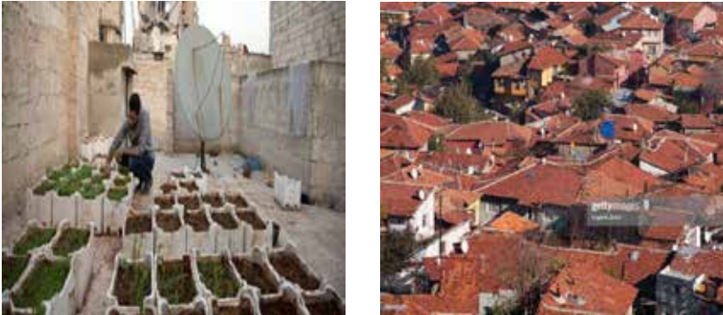
Figure 9: Flat roofs in Syria(Left), Pitched roofs in Ankara(right)
