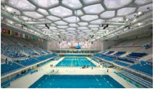
Figure 5: a)Water Cube Cephe Strüktürü b)Interior Space (“Designing the National Aquatics Center (Water Cube) for Beijing Olympics 2008 - Arup,” n.d.)
