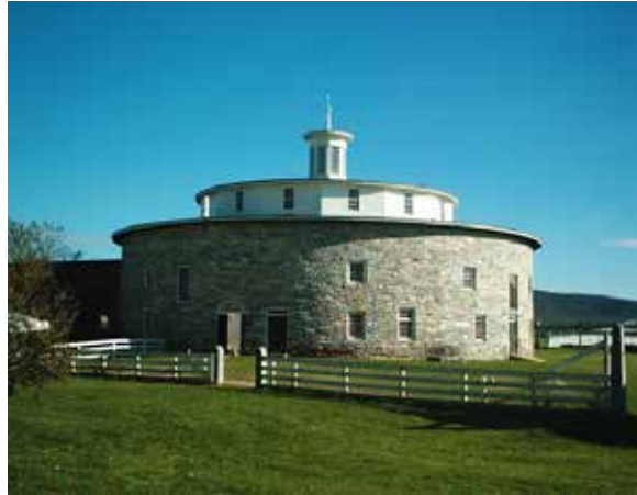
Figure 6: A Shaker structure, Hancock, Massachusetts, (Stein, 1994)
