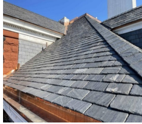
D. Slate roof
