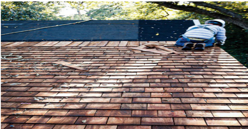
Figure 3. Wood shingle roof with cedar breathes
