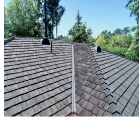
E. Concrete tiles roof
