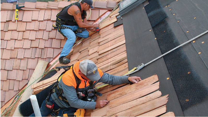
Figure 2. Wood shingle roof installations
